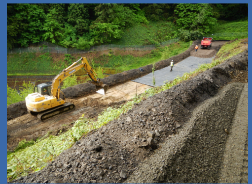
Preparation of onsite haul road
